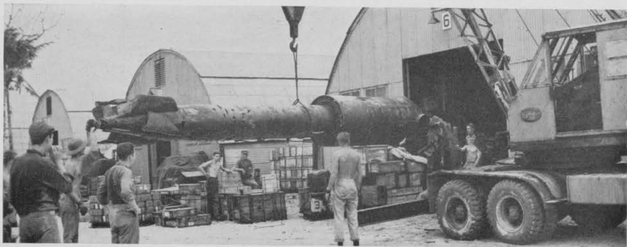
Human Torpedo, ULITHI Type—November 1944. Note cylindrical pilot's compartment forward.
